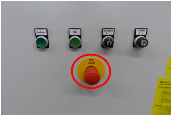
Fig. 50: emergency-stop push-button
