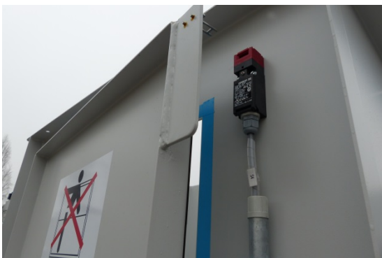
Fig. 64: safety switch revision door funnel
