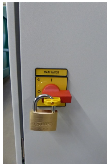
Fig. 13: master switch with locking device
