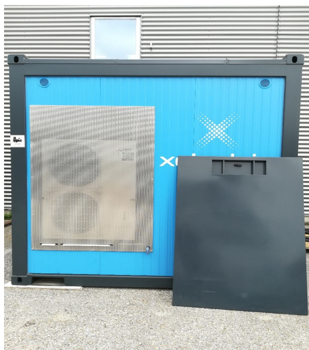
Figure 3: Transport protection for air conditioning system
