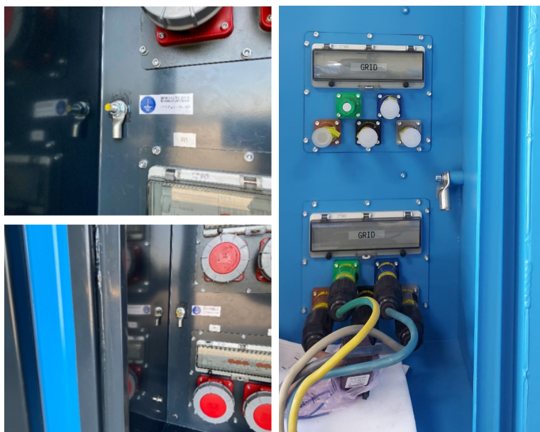
Figure 1: Earth Potential for the Unlimited M10 unit on the left and for the unlimited M20 on the right
